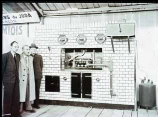
1922 - brick oven with direct intermittent heat
